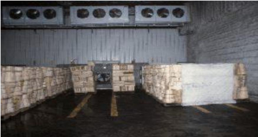
*Figure 2: A commercial forced-air cooling system.*
